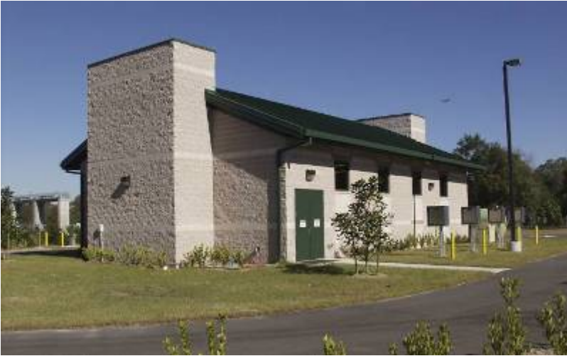
Tampa Bypass Canal
