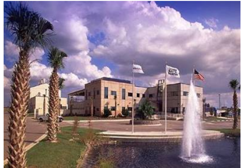
Regional Surface Water Treatment Plant
